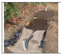
Typically the liner would finish about 100 mm below the surface and may be protected, for example by an old carpet.
