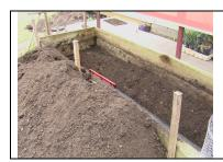
The base must be flat and a slotted drainage pipe laid to spread the water.
